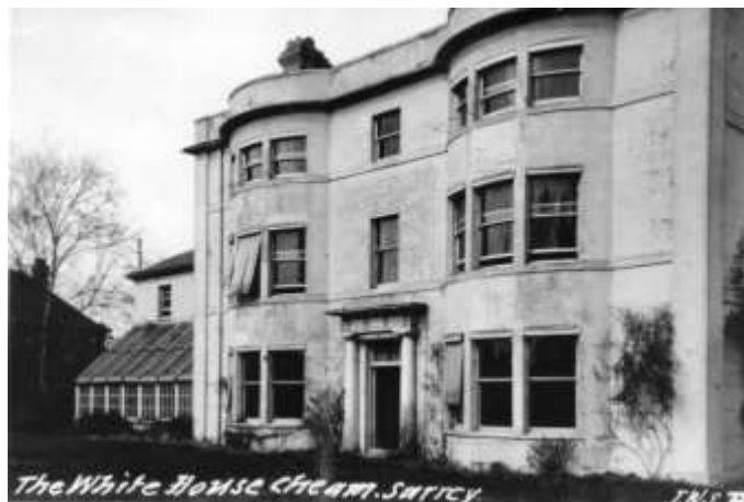
The White House shortly before its demolition. (Sutton Archives)
